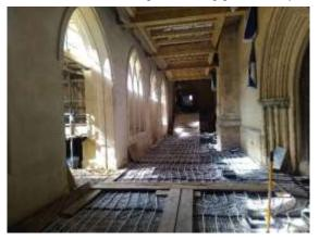
Work on the Friends Cloister Gallery is progressing with the ground floor underfloor heating installed and a Limecrete slab formed on top. The Purbeck stone of the floor is now being set out. The underfloor heating extends throughout the Cloister, joining up with the system recently installed in the Chapter House and extends all the way into what will become the new Cathedral Shop (below left).
